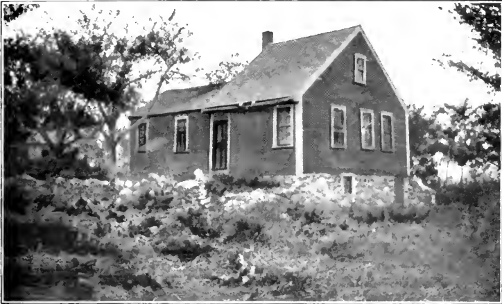
WEST END SCHOOL-HOUSE
